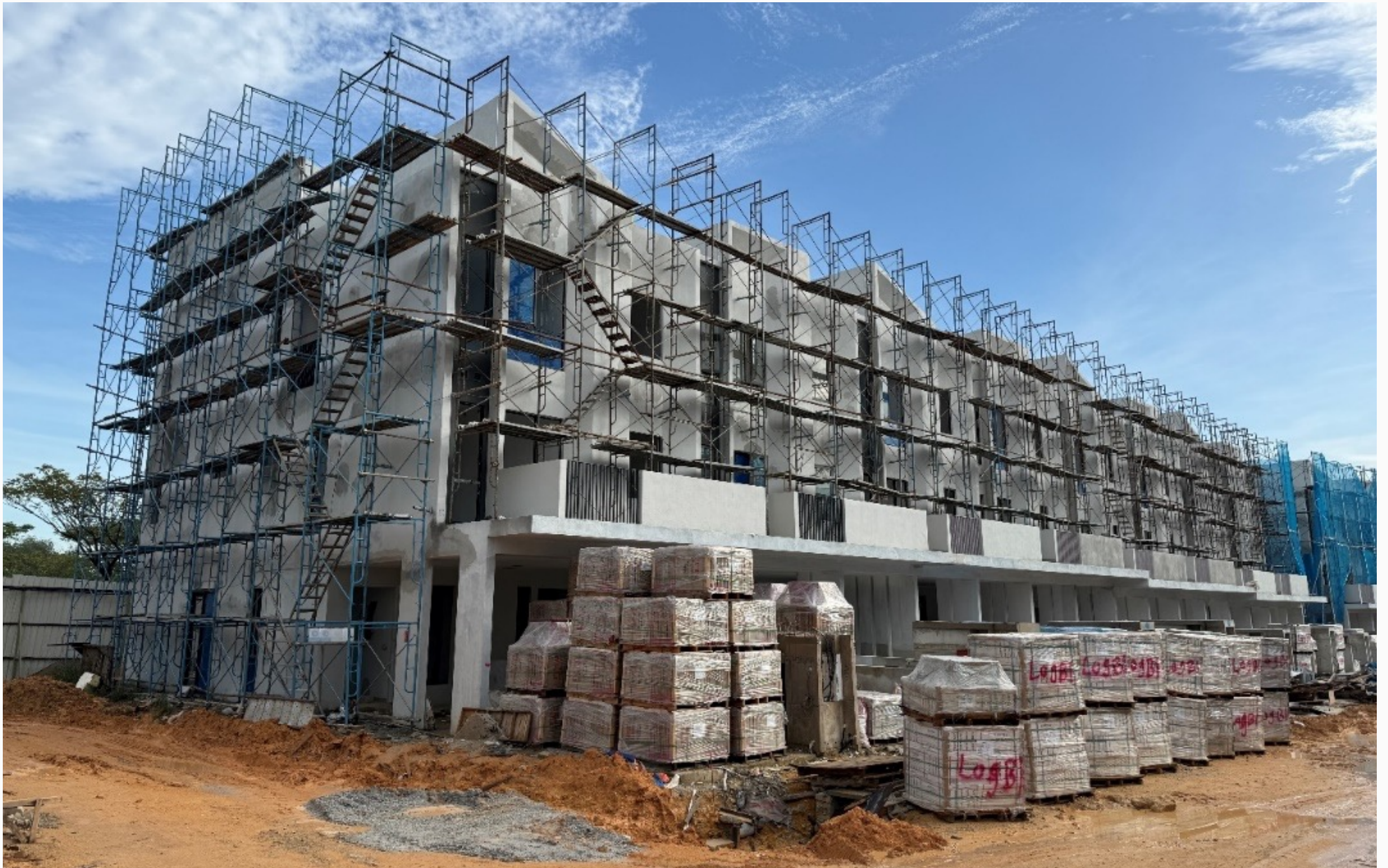
Townhouses (Row 1): External finishing works are in progress.
