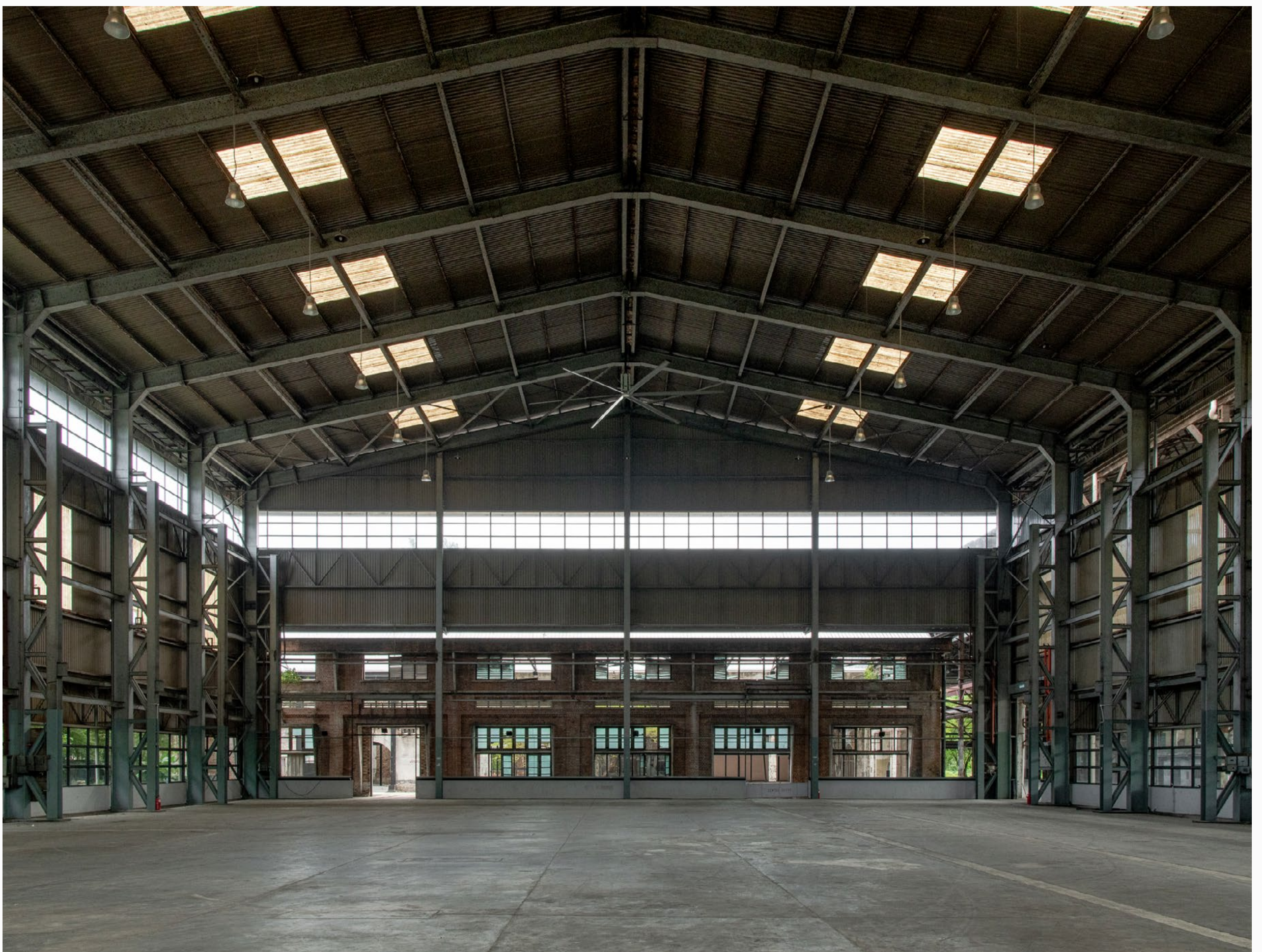
A surviving railway workshop at Sentul Depot was adapted and repurposed for new use as a versatile venue for lifestyle events while retaining the heritage significance of the space.
