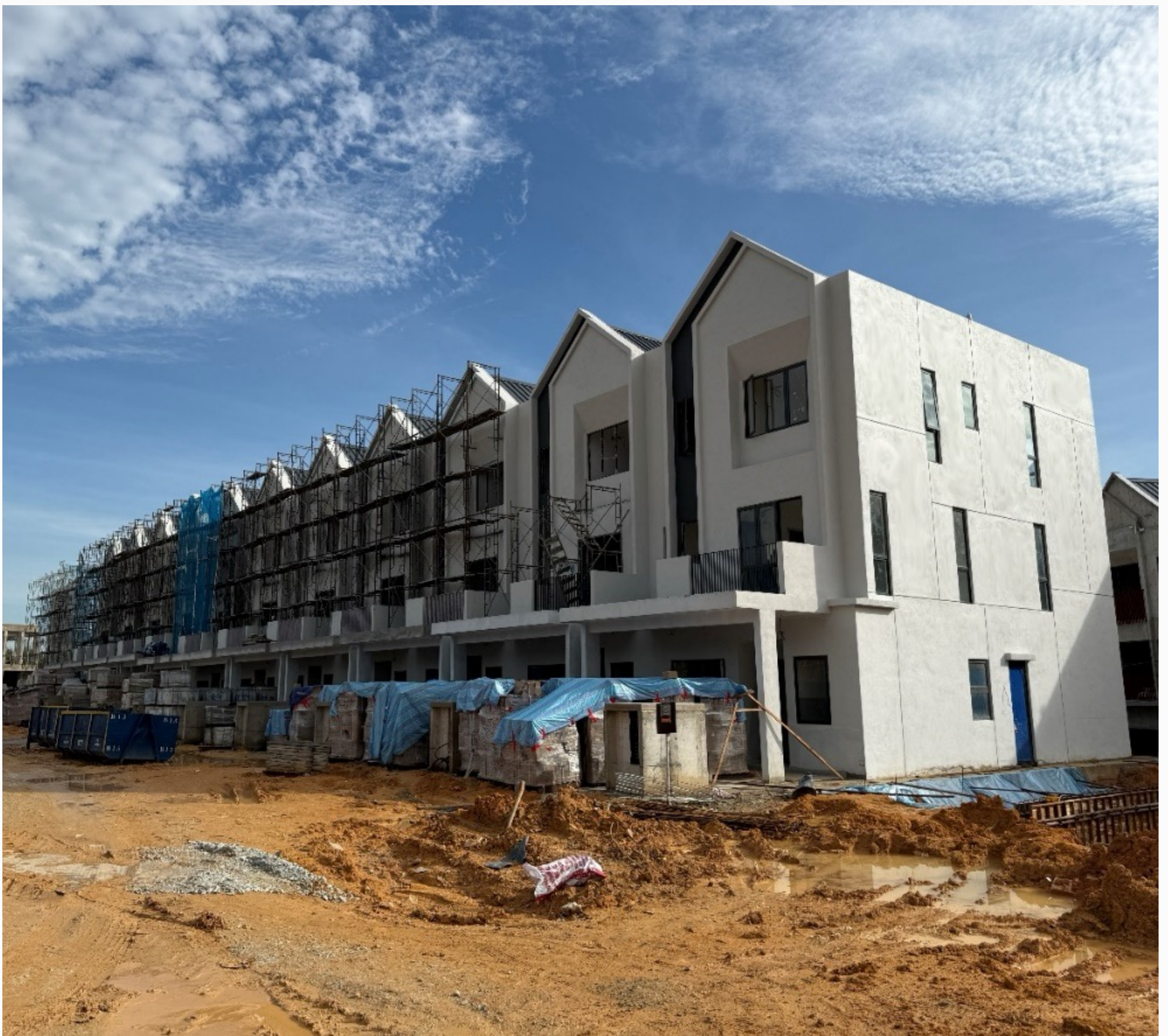
Link houses (Row 18): External finishing works are in progress.
