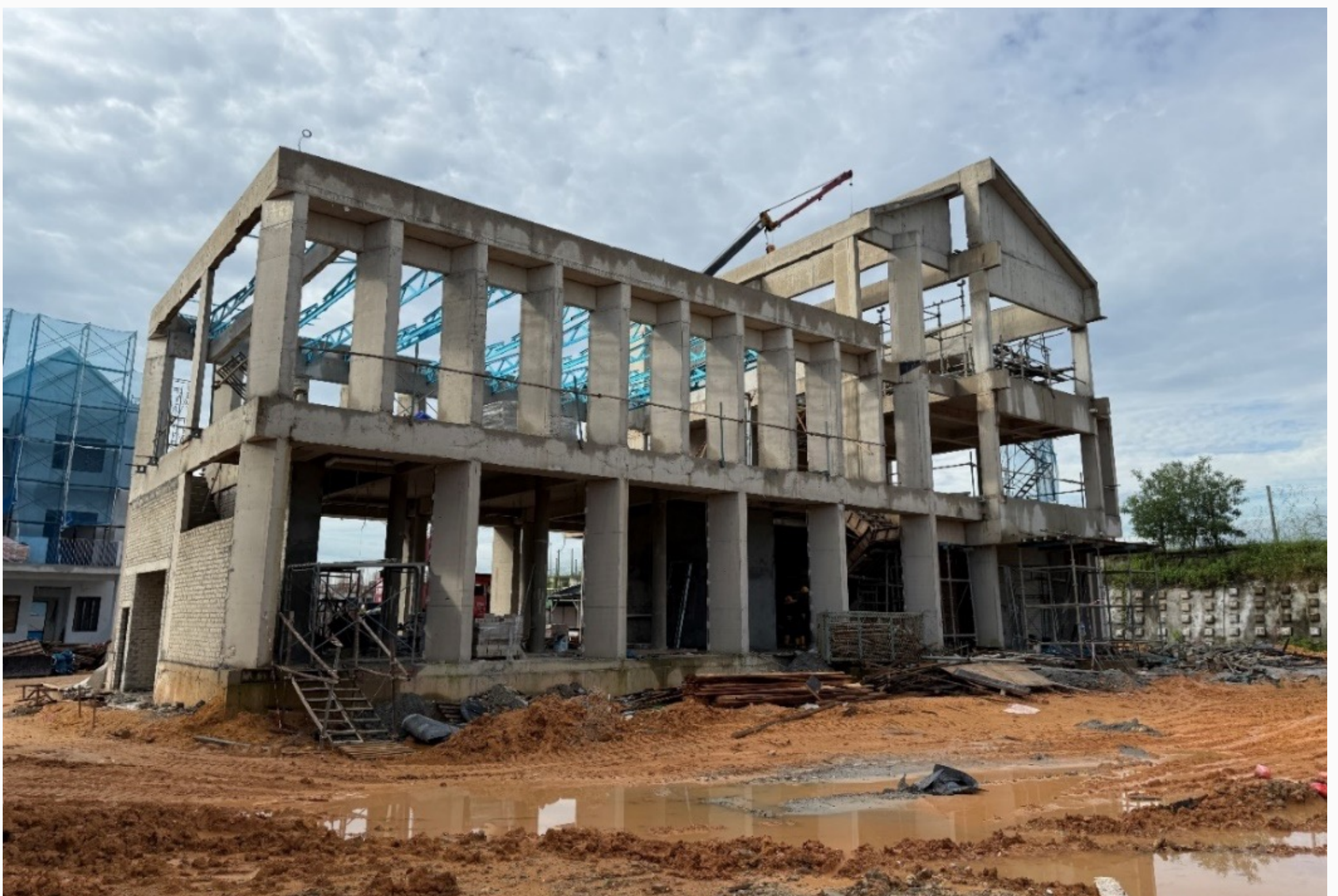
Clubhouse: Structural works and brickwork are in progress.
