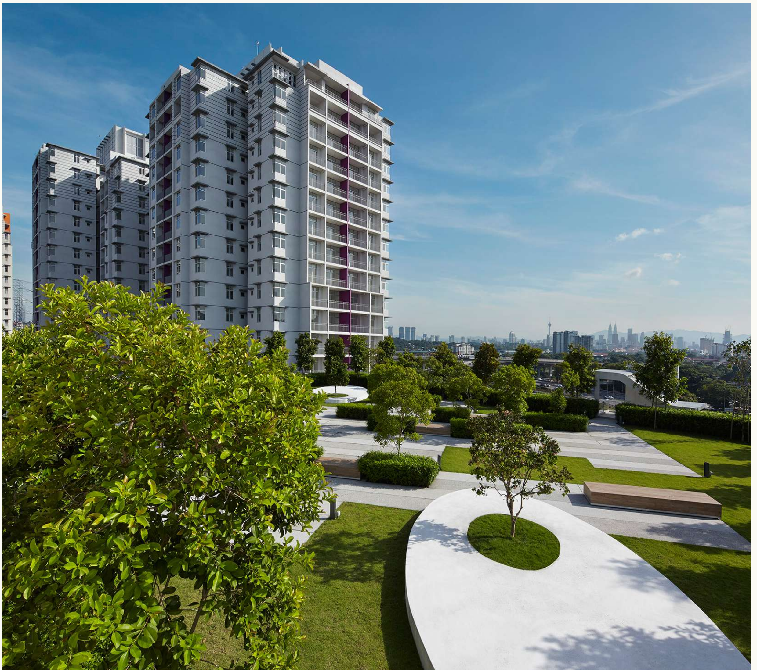
Exemplifying our desire to enhance with greenery wherever the opportunity exists, this podium carpark rooftop at Midfields 2, Sungai Besi has been transformed into a stunning open garden space for residents to enjoy.
