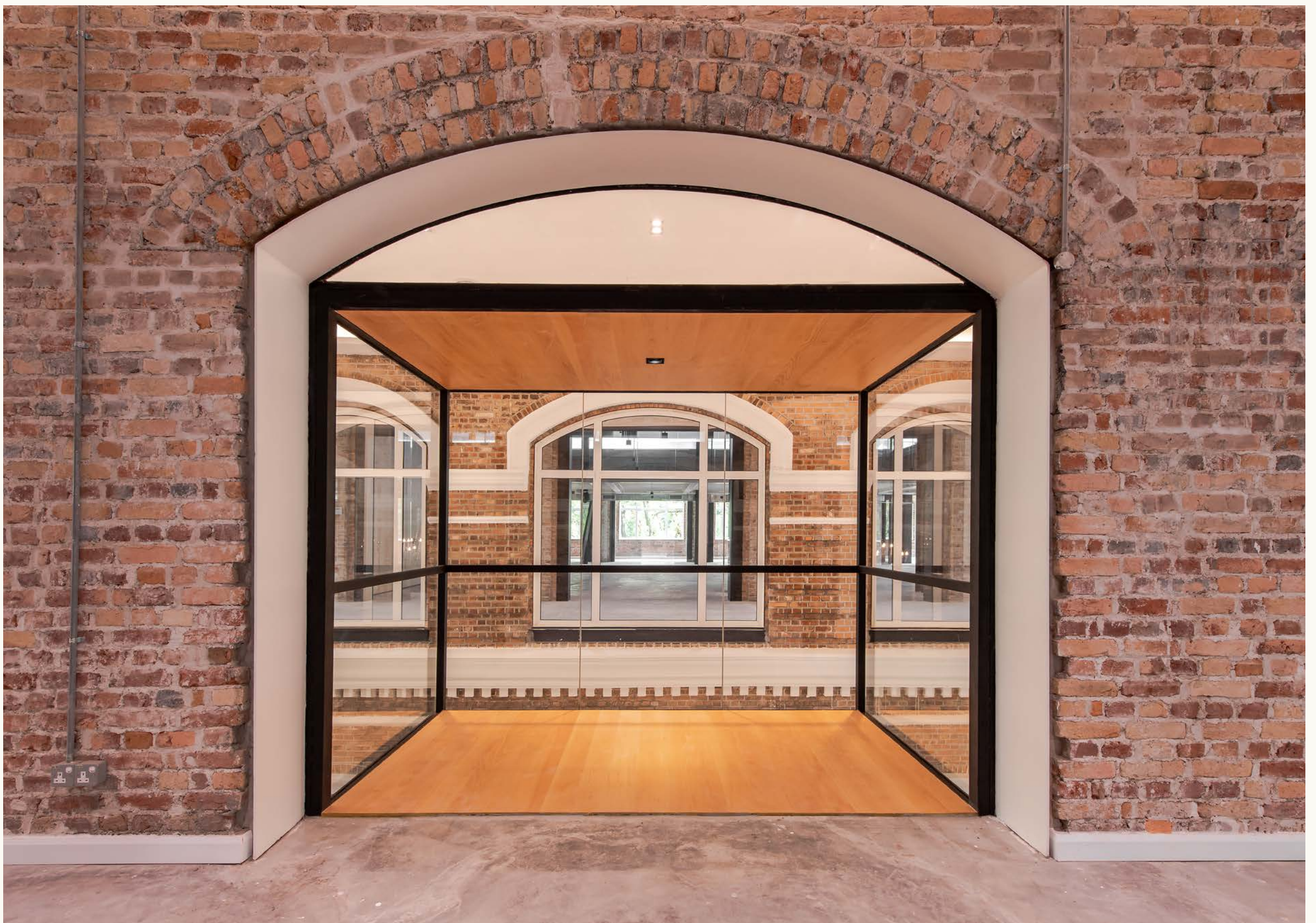
An eye-catching glass pop-up box hovers over the open space from the first floor.
