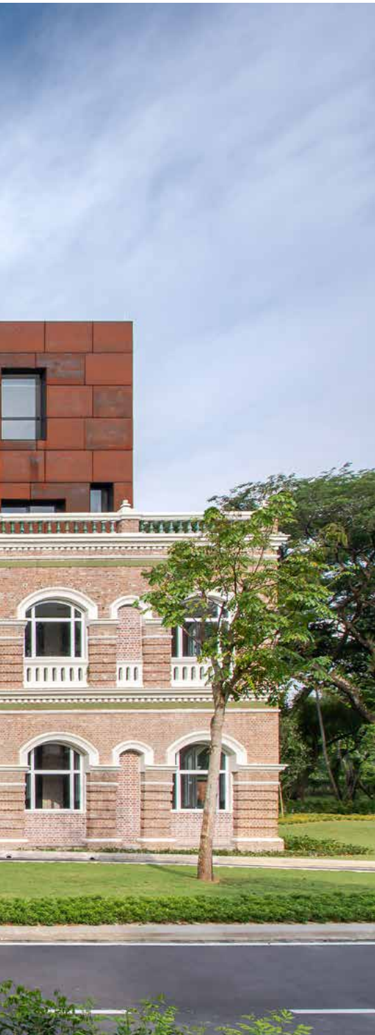
04. The material palette of oxidised Corten steel and weathered timber-strip decking lends a rustic character to the scheme, offset by the precision of glazed façade and variable panel widths of cladding.
